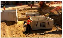
Vault Oil Containment kits are custom designed to capture any leakage from underground transformer vaults. The containment consists of a prefabricated unit featuring four oil immobilizing mats secured between two layers of impermeable liner in specifically chosen locations and size to maximise drainage without sacrificing performance. The
